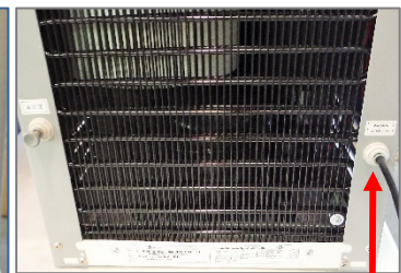
Water Supply Line
