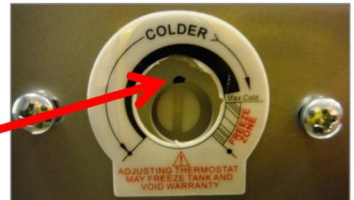
Turning the adjustment screw clockwise to lower the set point temperature.
